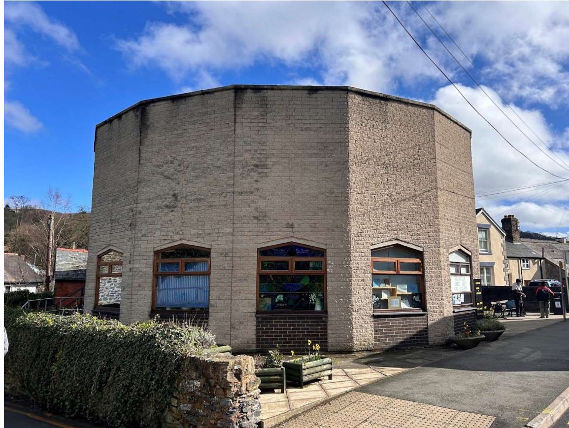
View North-Eastwards towards existing front elevation
