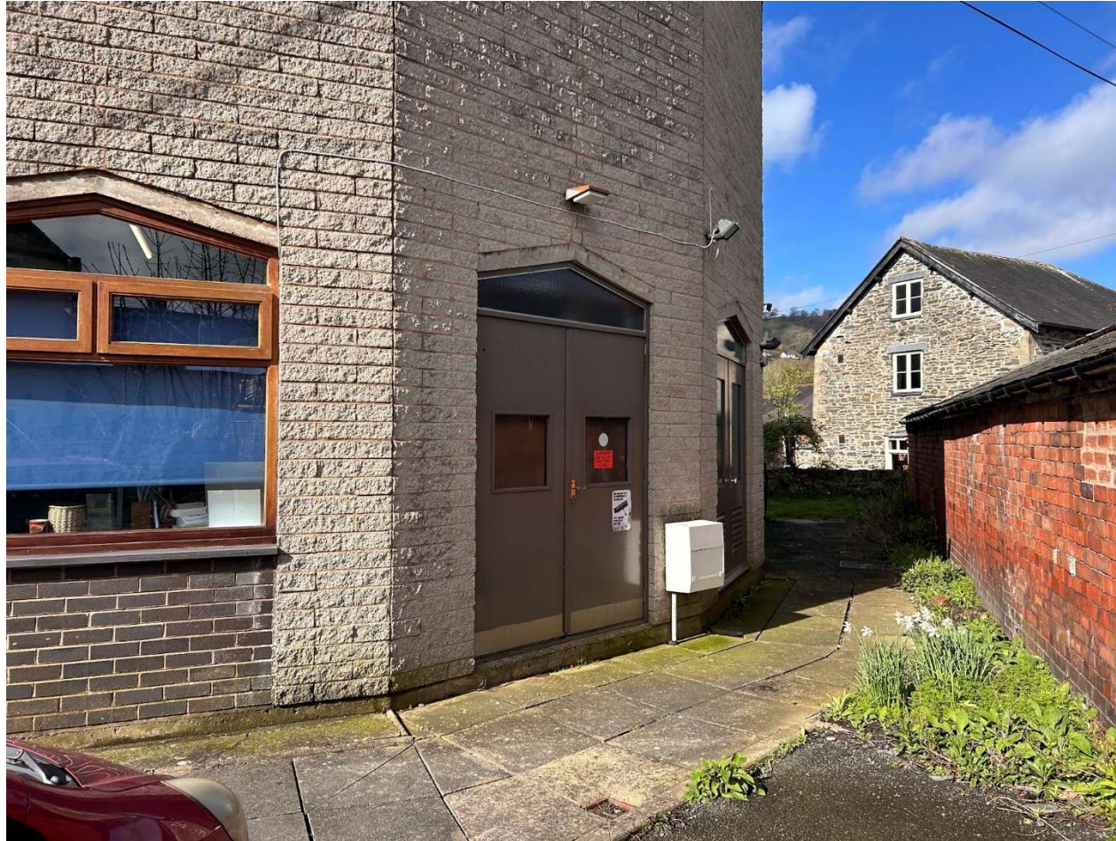
View Westwards along rear elevation
