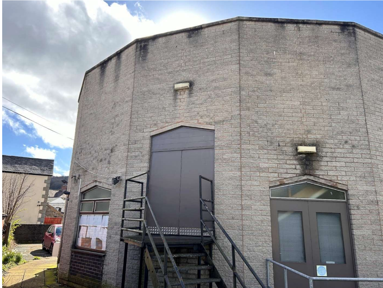
View Souht-Eastwards towards existing rear elevation
