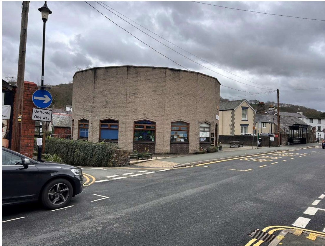
View North-Eastwards towards existing front elevation
