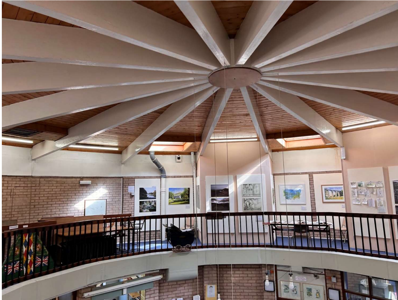
Internal view of existing roof structure
